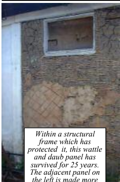
Another method using building rubble trapped between a framework of bush poles and bamboo laths has proved equally durable.
