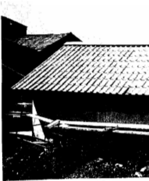
EXAMPLE OF ROOF
