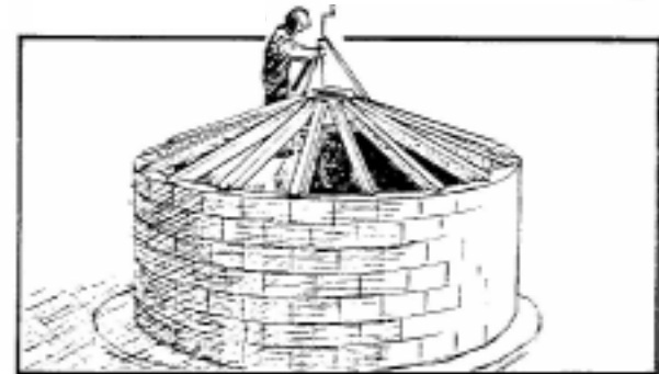
6. 18 beams are fitted in position the jack is removed.
