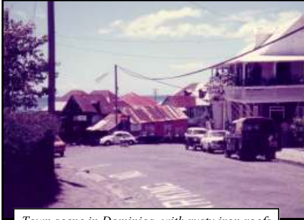
Town scene in Dominica, with rusty iron roofs (Photo: J Parry)
