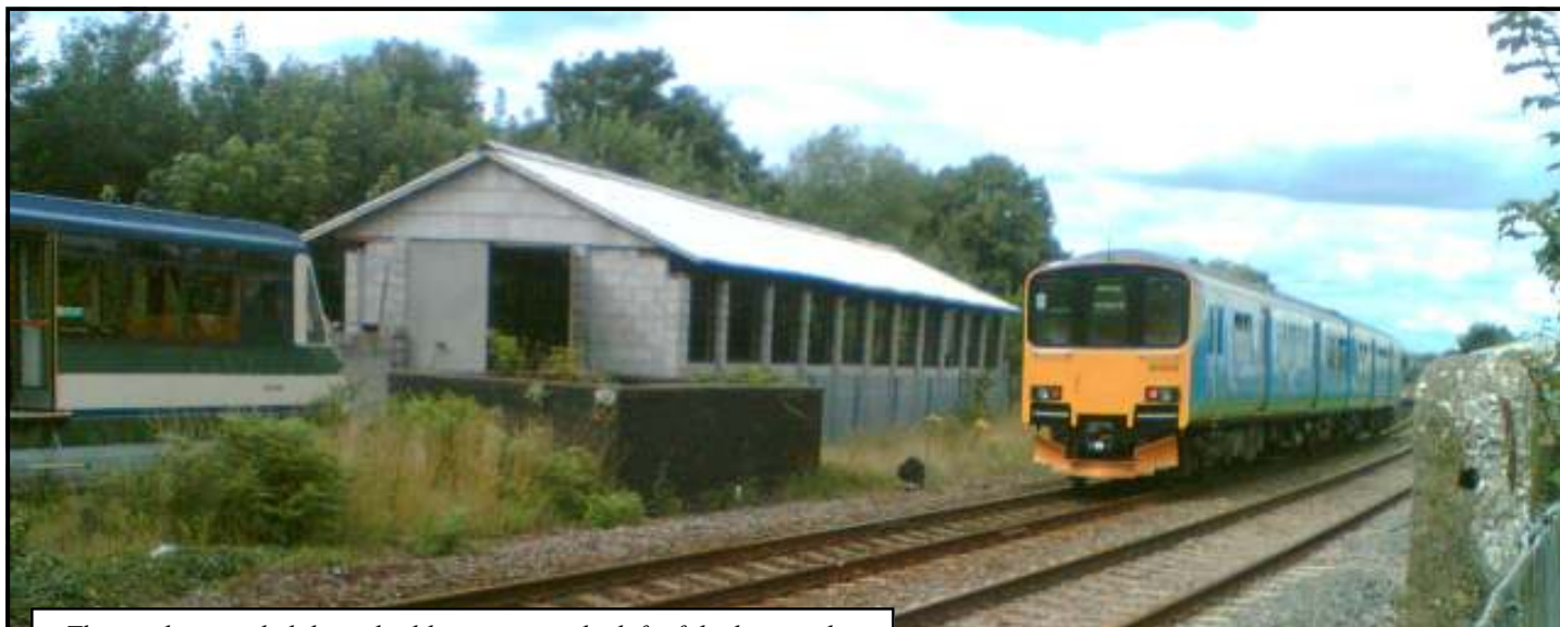
The newly extended depot building seen on the left of the line, with a main line train (inbound from Worcester) on the right of the picture
