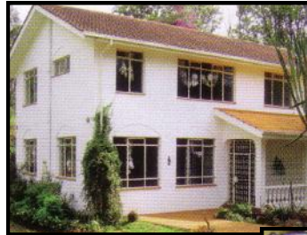
Conventional construction in Kenyan residential housing.
